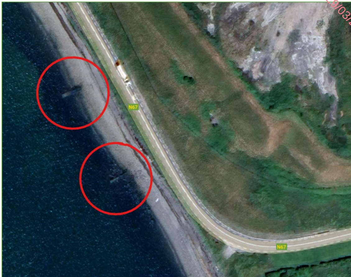
Image 3.1.2 – 2No. culverts discharging to the bay adjacent to the N67
